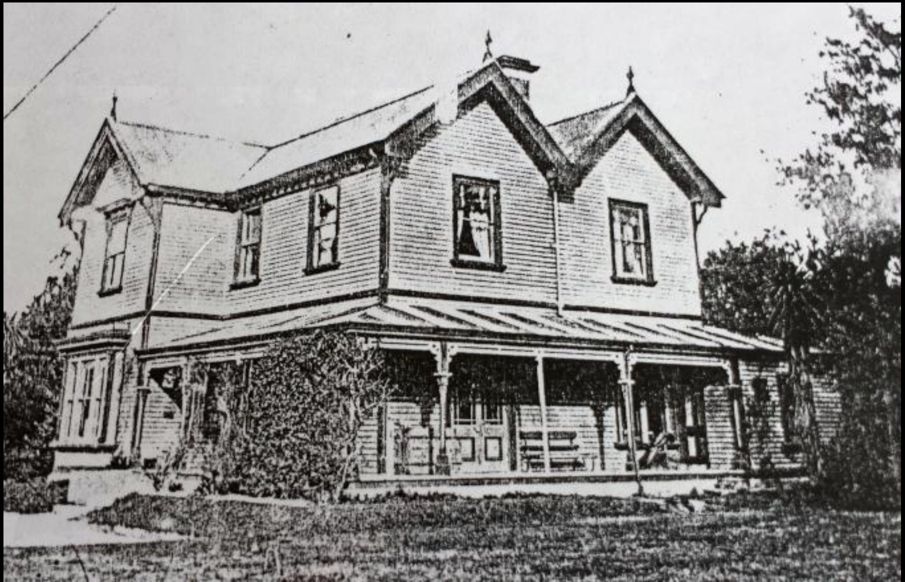
Fendalton Vicarage built on glebe land near the Waimairi Stream in 1886
